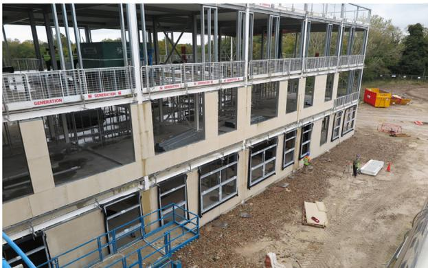
External cement boards and windows are now installed on much of zone 4
