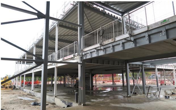
Steel metsec is being progressed across zone 2, which will allow for the cladding to be installed.
