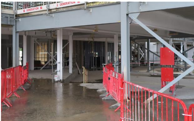
Internal spaces take shape in zone 3 through internal partitions. Mechanical & Electrical works are also commencing.
